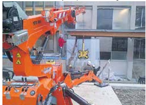
Glass installation is safer and more efficient with this Jekko SPD360 and its specialized attachments.
